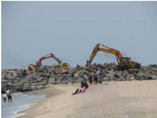
Figure 11. Construction of a groyne on Karraikal beach
