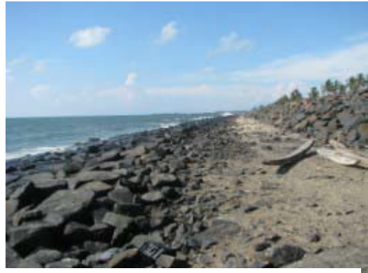
Figure 10. Seawalls on Puducherry beach
